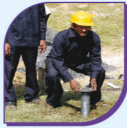
Inserting Electrode Step 2 →
